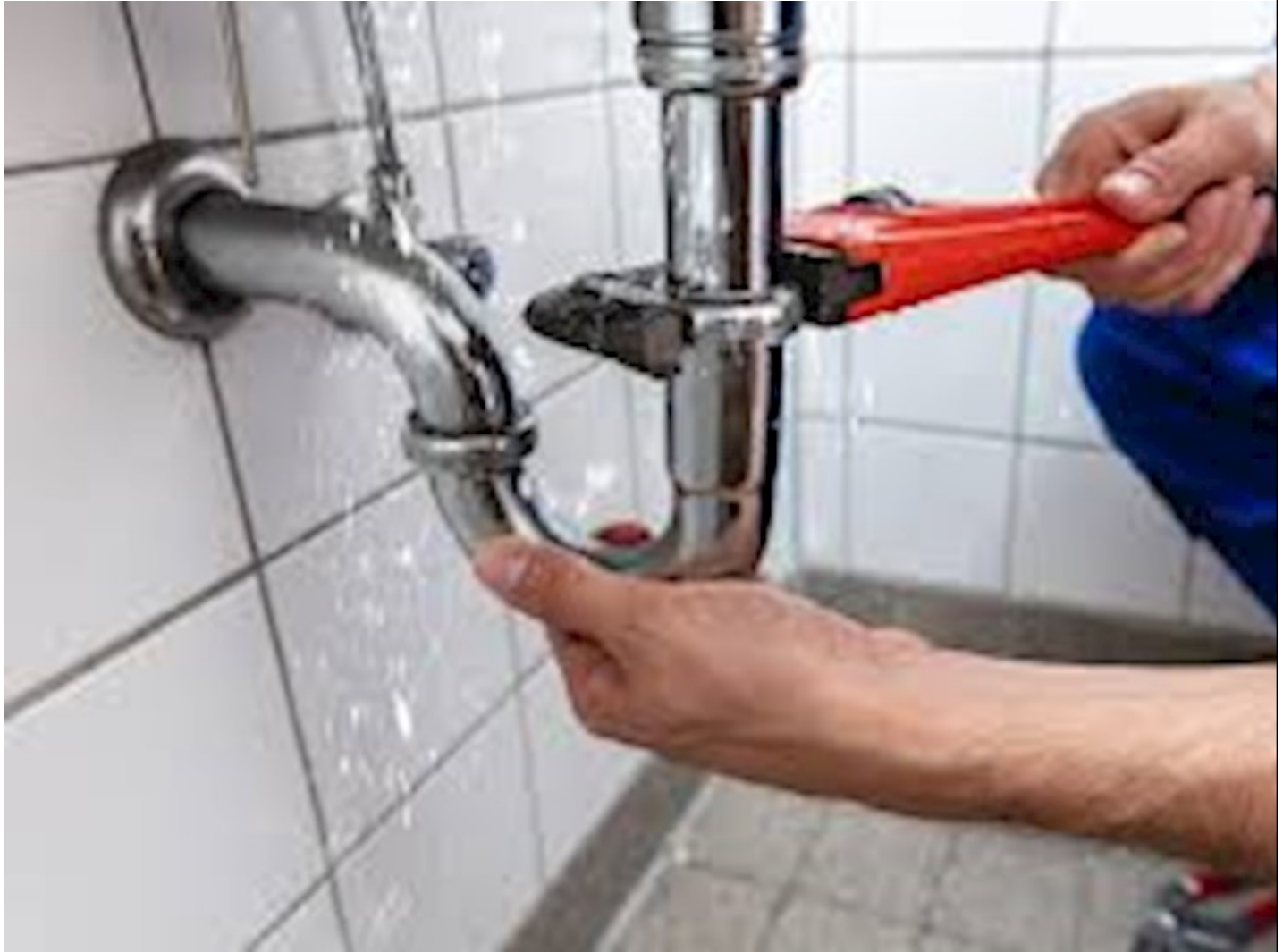
Photo – Plumbing Bathroom 1
